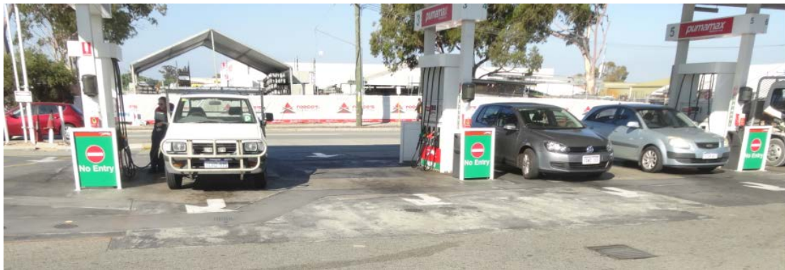
Puma 502 Guildford Rd, cnr Katanning St, Bayswater. 'No entry' signs to bowzers as viewed from the Guildford Rd crossover side of the development. Marked arrows directing customer vehicles to exit the site onto Guildford Rd.
