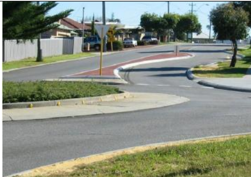
Figure 19 - example of a roundabout pre-deflection
