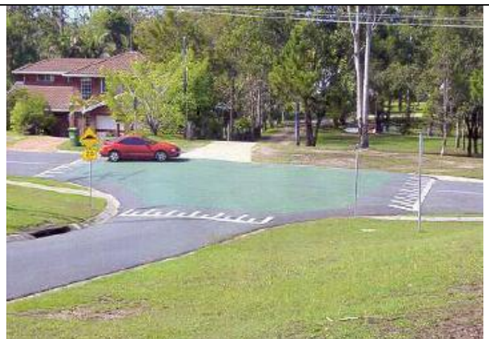
Figure 14 – example of intersection coloured surfacing
