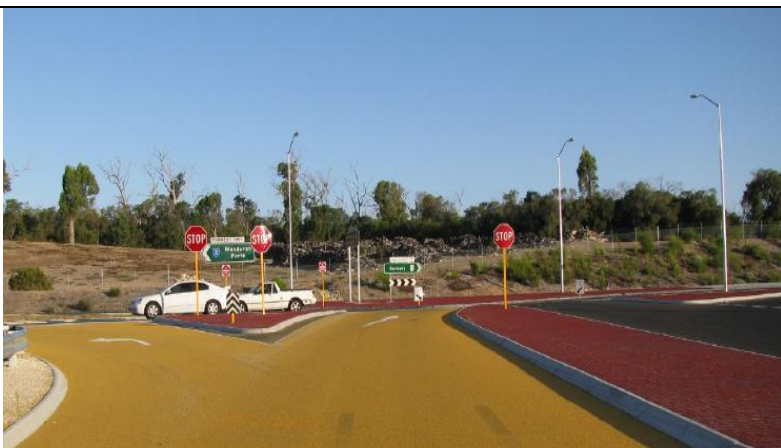
Figure 13 - example of intersection surface treatment
