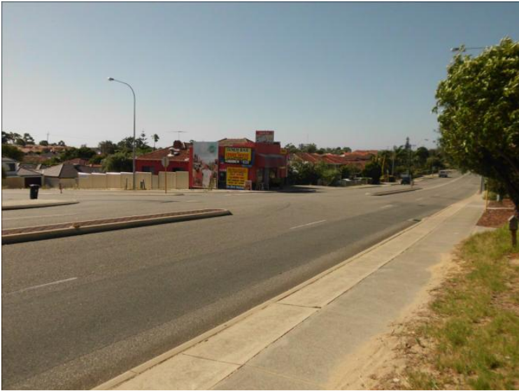
Figure 11 - existing median treatment at intersection
