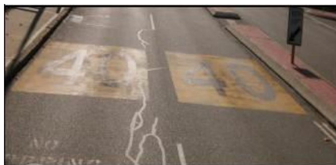
Figure 22 – speed pavement markings
