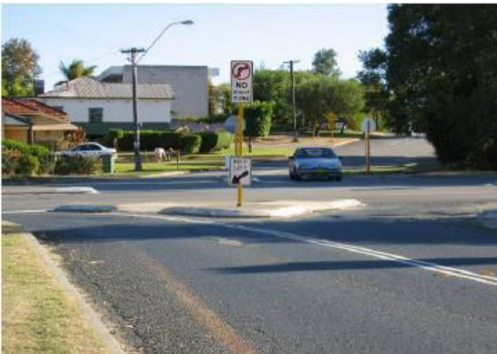
Figure 17 – example of left in left out intersection
