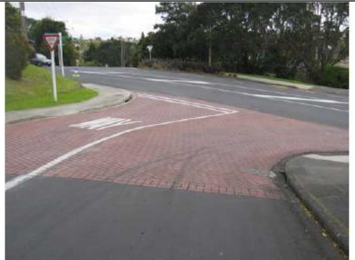
Figure 16 - example of intersection threshold treatment
