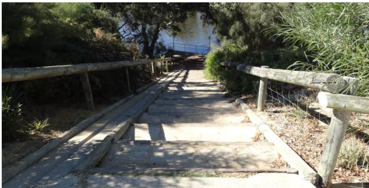
Figure 5-8 Stairs connecting the riverside path to Ashfield Parade
