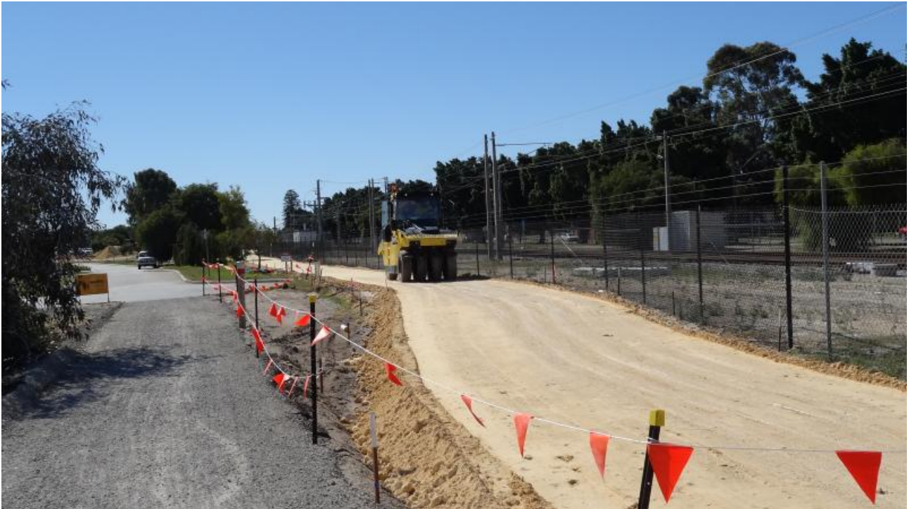
Figure 5-4 Midland Train Line PSP under construction in Bassendean (May 2012)
