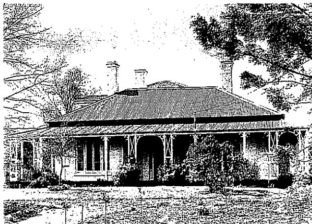
△ 66 Fernleigh, Midland Highway, Kempton, Tas. Architect and date unknown. The encircling veranda features timber trellage.
