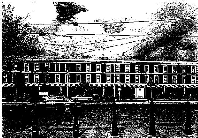
△ 65 Royal Terrace, Nicholson Street, Melbourne, Vic. John Gill, architect (attrib.), 1854-56. Dignified row houses in a once-fashionable residential address.
