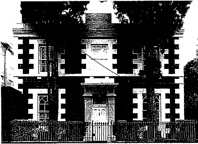
△ 64 House, Hanover Street, Fitzroy, Vic. Built by Edward Wills, stonemason, 1854. Intractable basalt expertly refined by moulded details.
