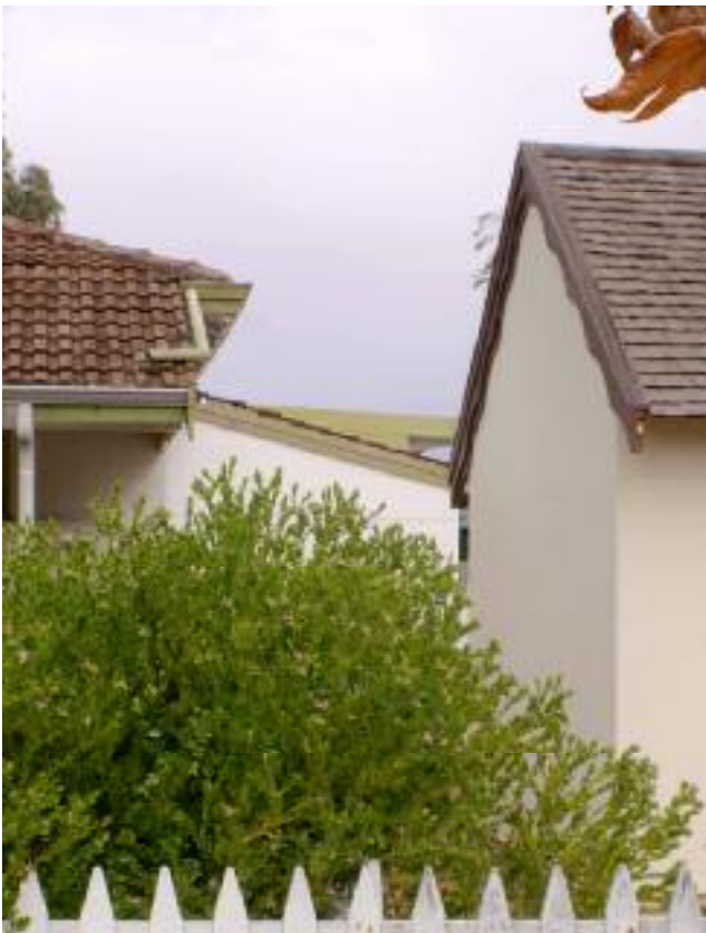
Photo 12 1 Surrey Street, Bassendean View looking south showing proximity of the residence, and the east gable wall. L Gray 7 June 2007
