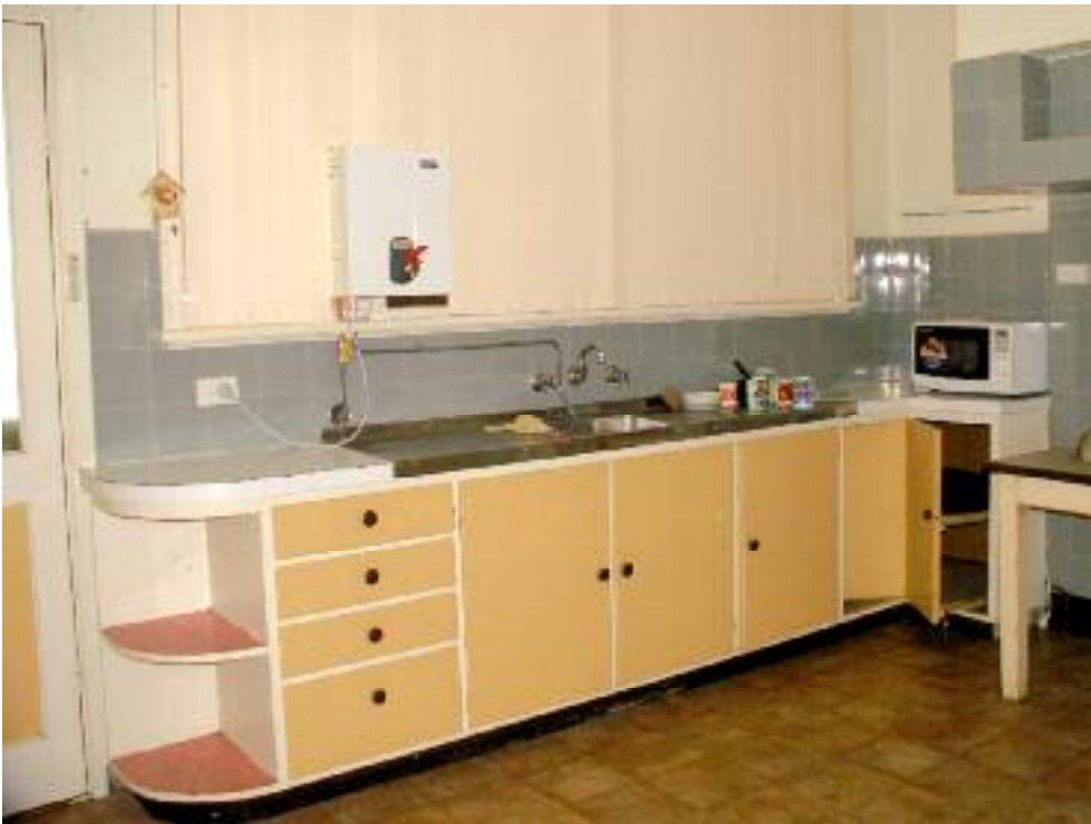
Photo 49 1 Surrey Street, Bassendean c.1952 addition: rear wall of kitchen, showing original fitout. L Gray 7 June 2007
