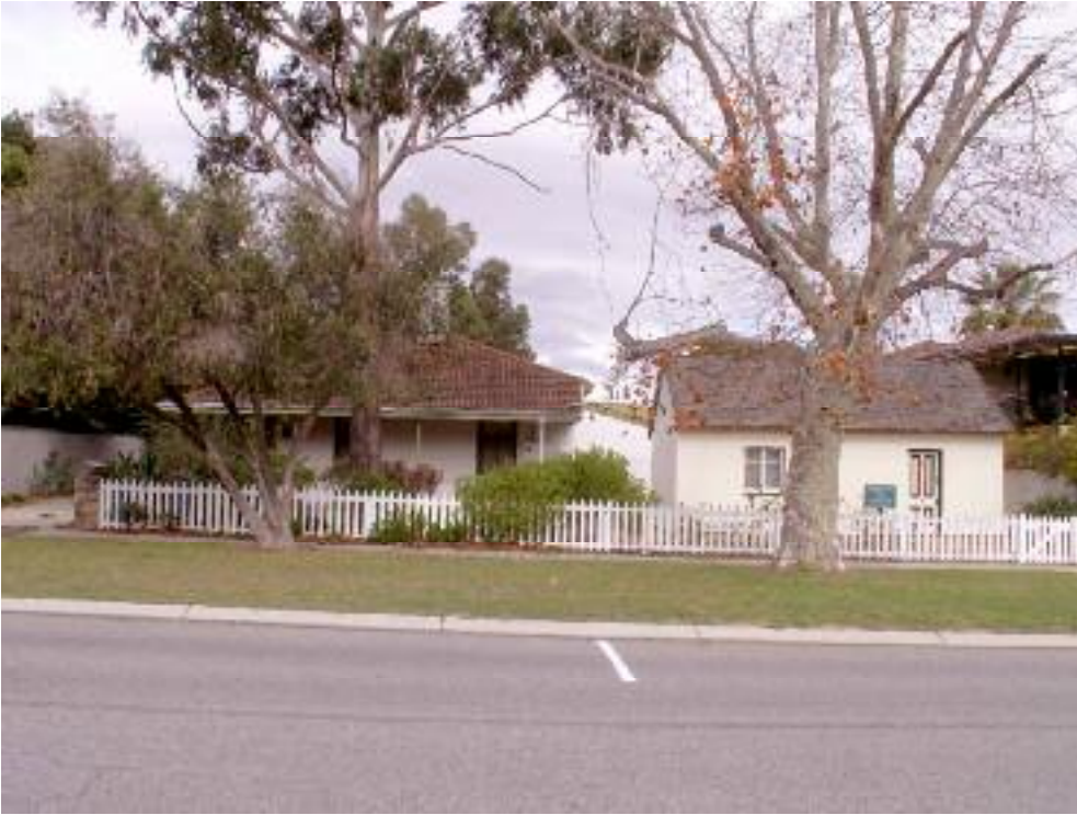
Photo 1 1 Surrey Street, Bassendean Streetscape view of north elevation showing Pensioner Guard Cottage (right) and c.1893 Residence (left). L Gray 7 June 2007
