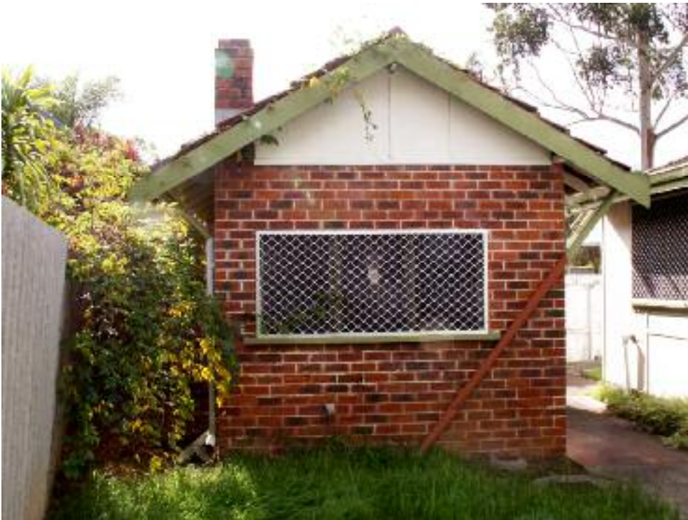
Photo 56 1 Surrey Street, Bassendean c.1952 laundry: south elevation. L Gray 7 June 2007
