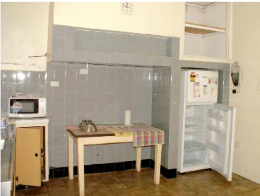
Photo 50 1 Surrey Street, Bassendean c.1952 addition: west wall of kitchen, showing original tiled recess. L Gray 7 June 2007
