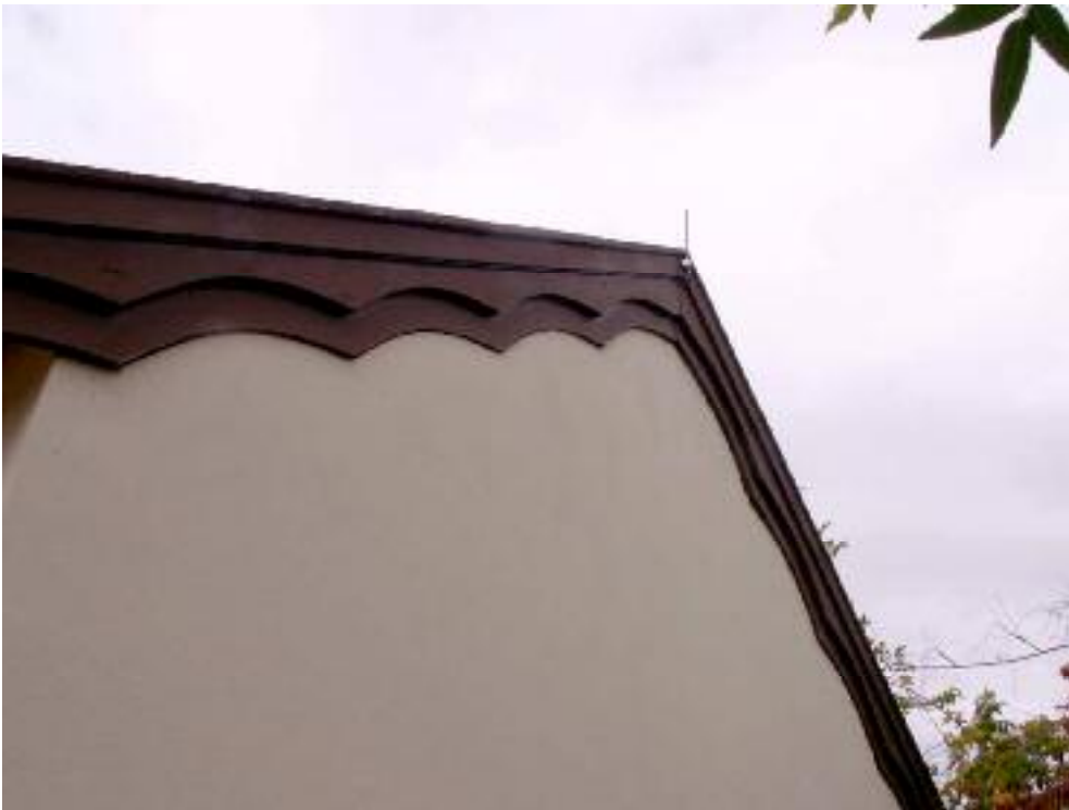
Photo 13 1 Surrey Street, Bassendean Detail of the reverse scalloped bargeboards. L Gray 7 June 2007
