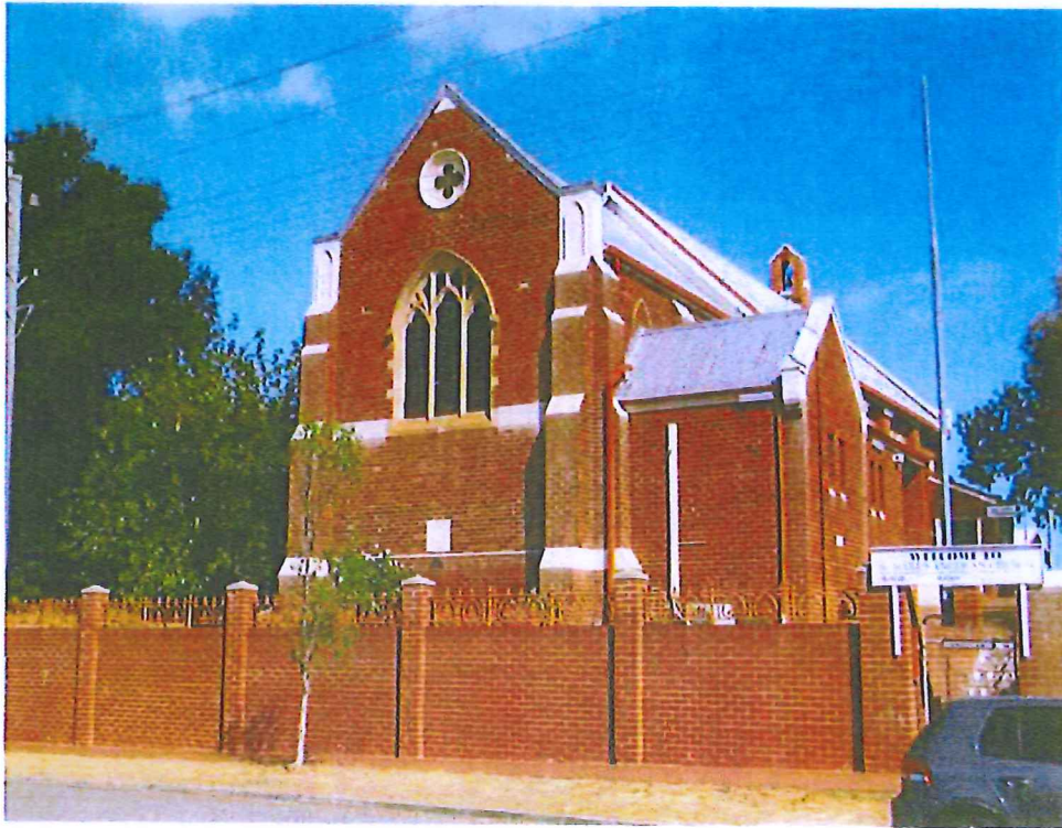
1. Eastern elevation to the street.
