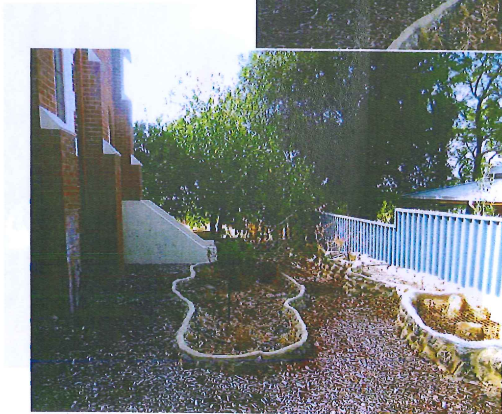
21. View looking east along the south side of the Church.
