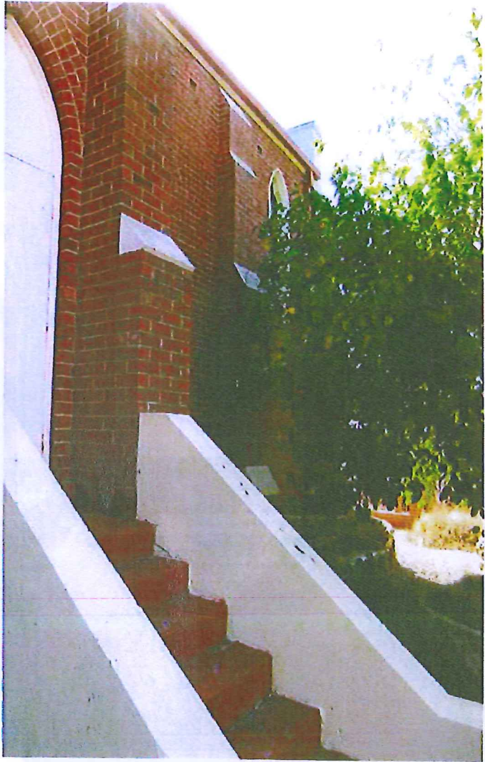
13. South elevation at the east end.
