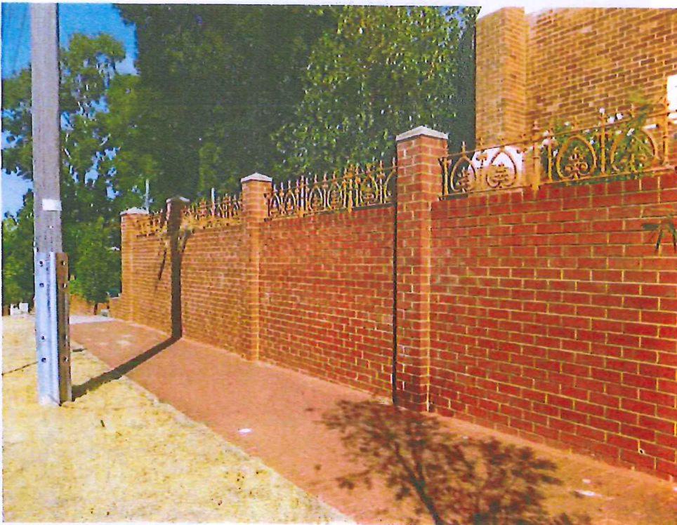
6. Retaining wall to the street.
