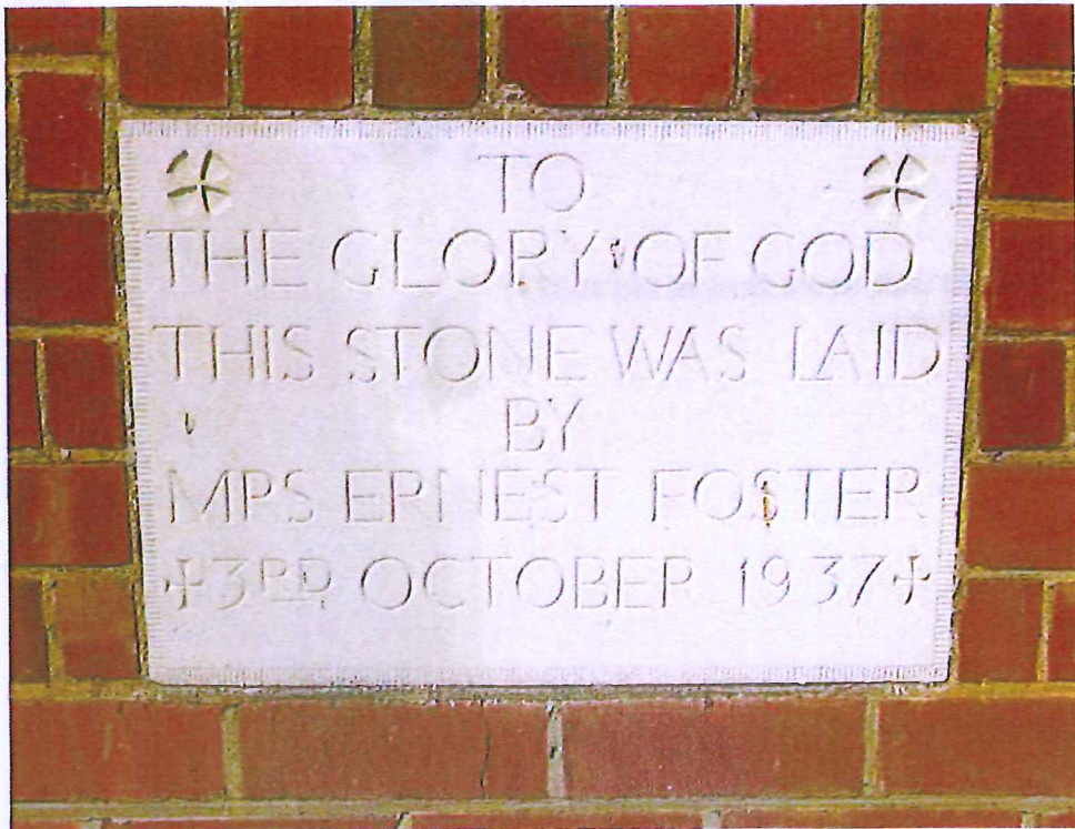
17. Foundation stone to the nave of the Church – north wall.
