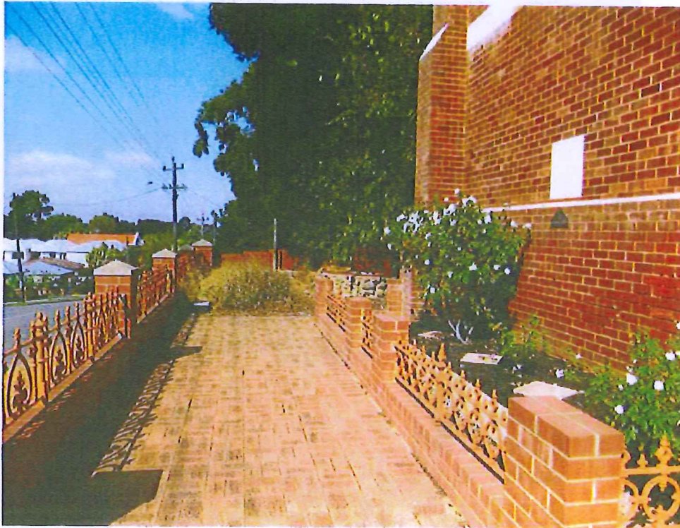
5. View south along the east wall of the Church.
