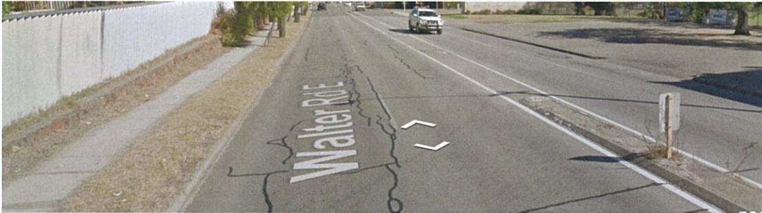
Figure 7: Walter Road East in the vicinity of the subject site - Looking west
