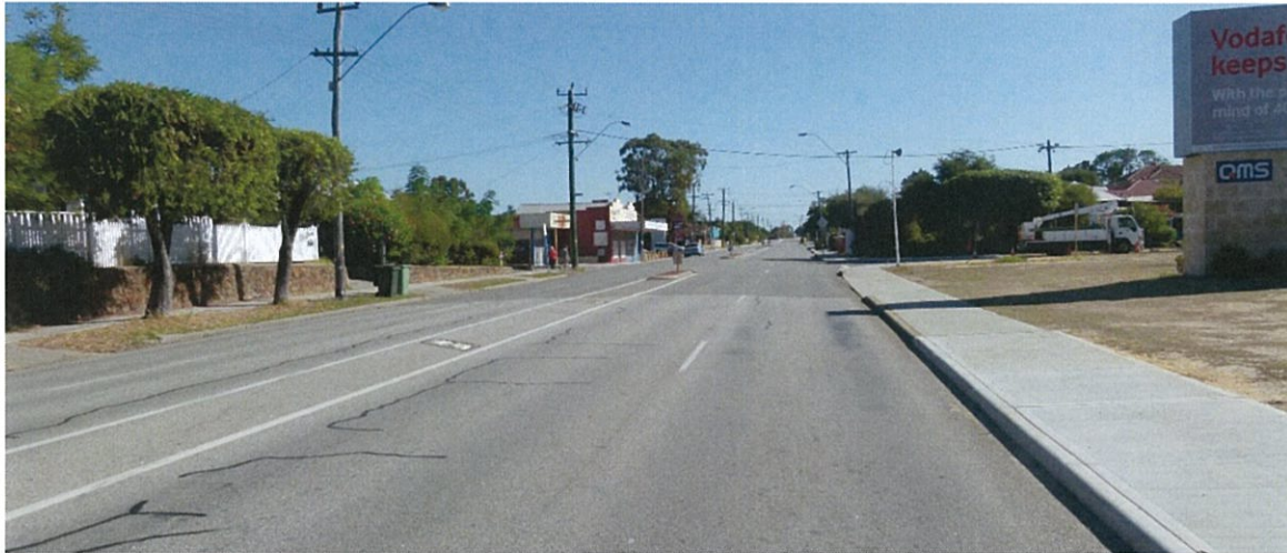
Photograph 4 – Walter Road East, as viewed from the subject site looking west.
