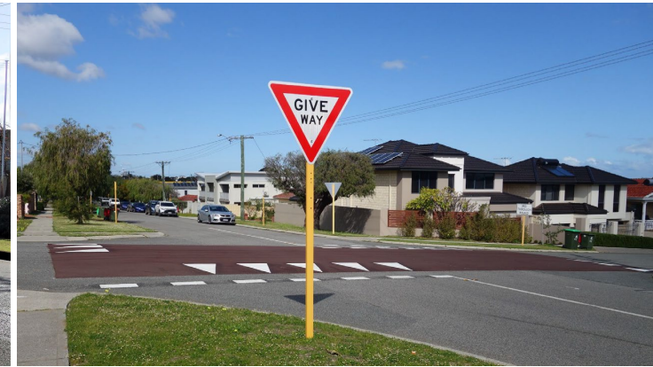
Joondana Raised safety platform
